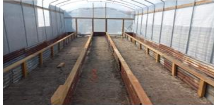
Raised planting boxes constructed for above ground cultivation
