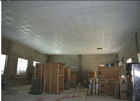
Construction of agro-processing factory.
